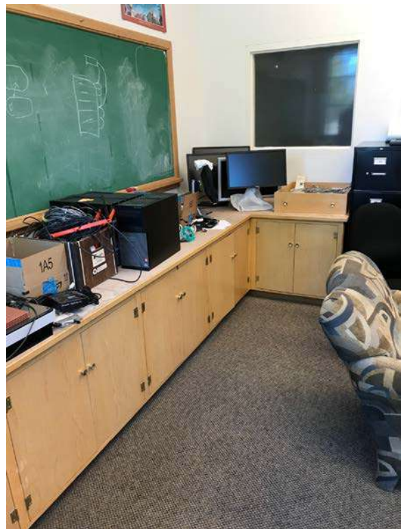
View of Room 180 Cabinets to be removed with ACM floor tiles beneath – chalkboard also to be removed
